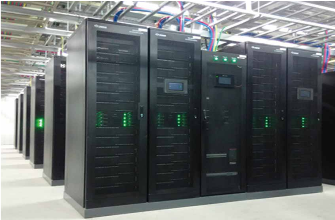
China mobile (Harbin) data center, 336V200Ah lithium battery system
