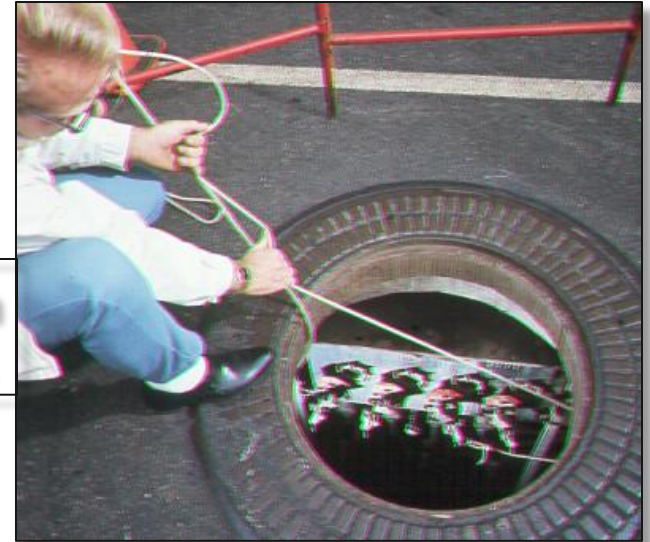
Typical wet vault or sub surface switch Vaults are under the street or sidewalk
