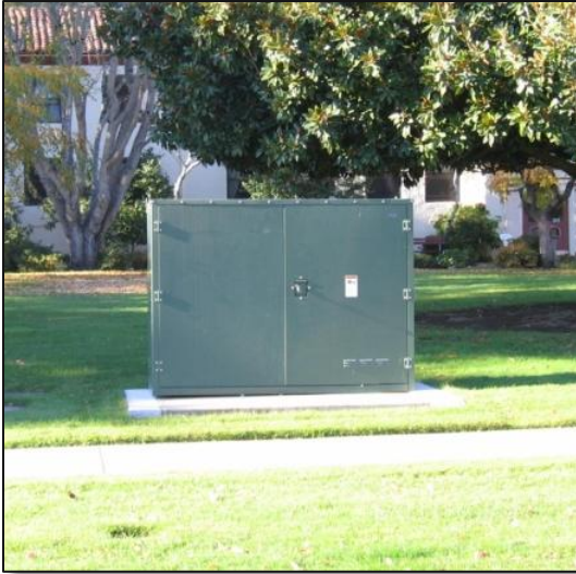
Typical pad mount switch Green enclosure mounted in the public
