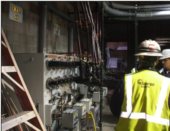
Typical dry vault or equipment room switch Found in basements or dedicated buildings
